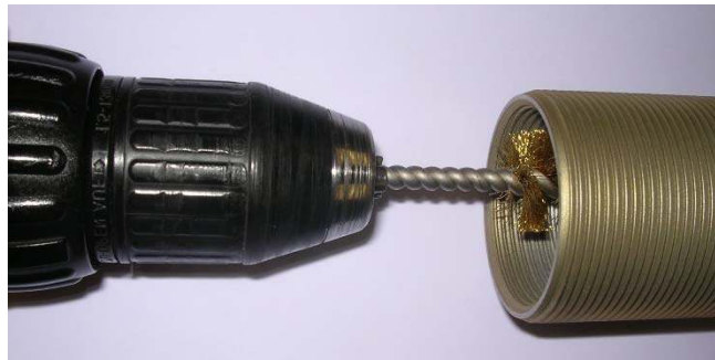
Pictures of brush cleaning of a stud
