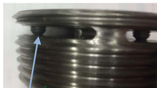
Pressed against Opposite Surface. No Gap.
