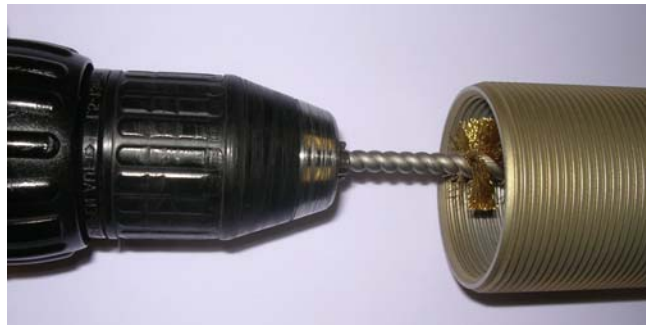
Pictures of brush cleaning of a stud
