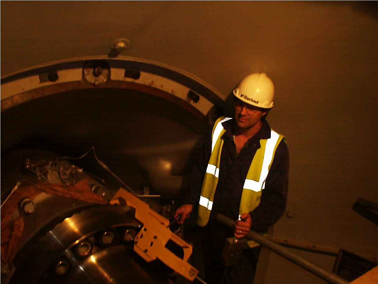
Photo 5 Tensioner in operation while mounted on 9FA turbine flange.
