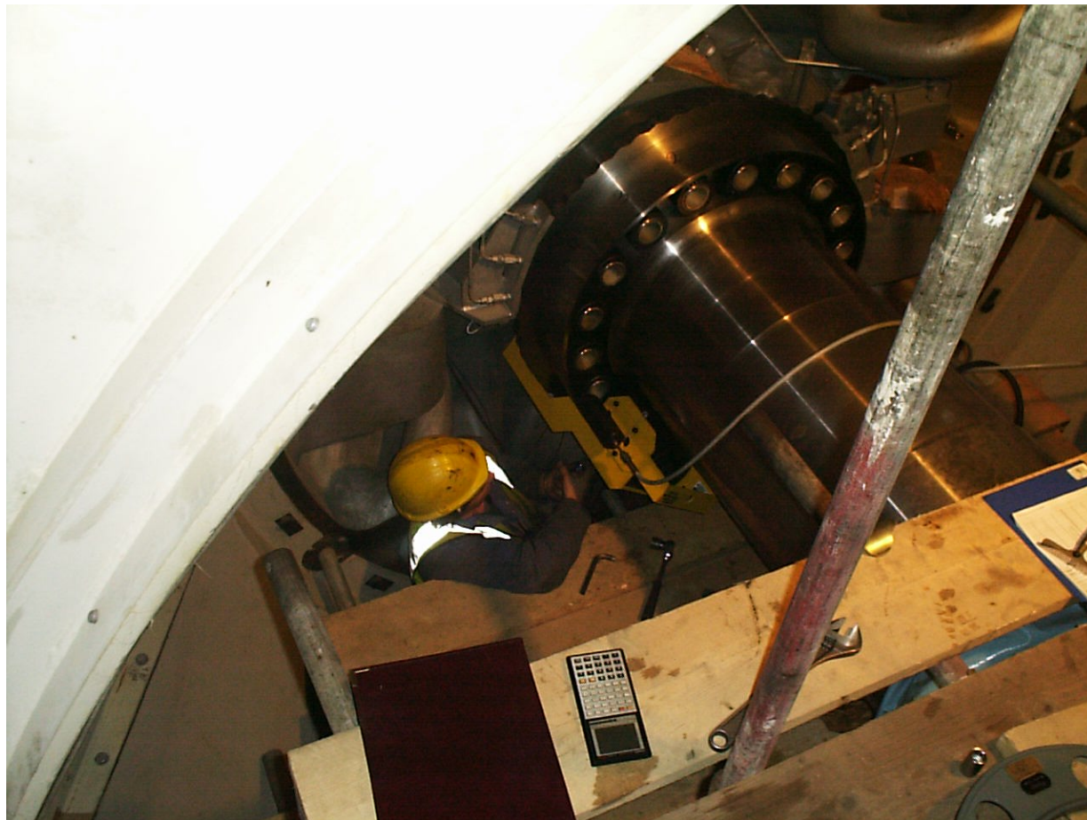
Photo 4 Tensioner in operation while mounted on 9FA turbine flange.
